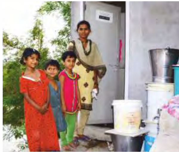
Beneficiaries with the toilet constructed by Shelter
