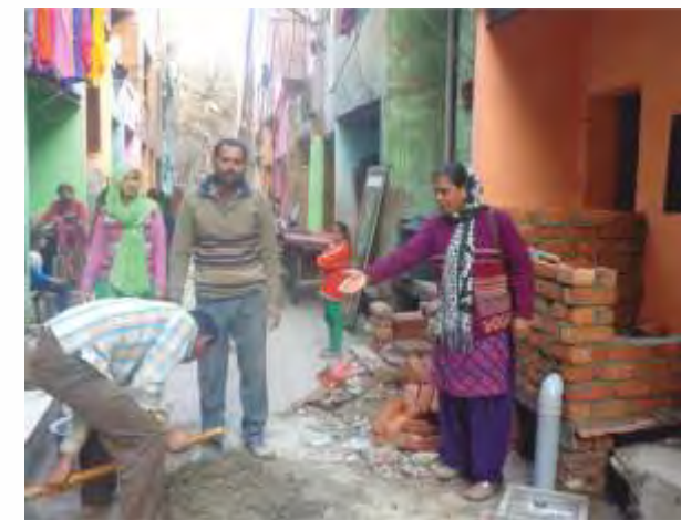
Under-construction toilet by MHT in Delhi
