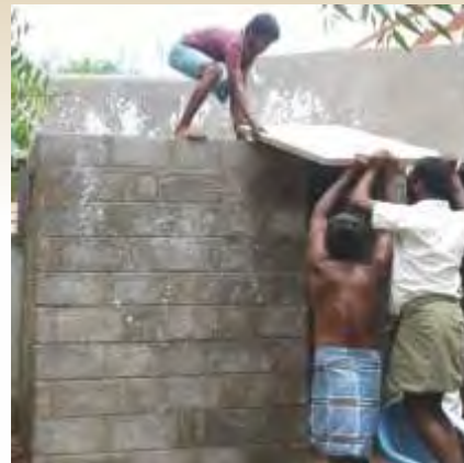
Under-construction toilet by Gramalaya in Trichy
