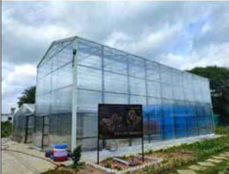
Processing Unit at the UPPAL FSTP
